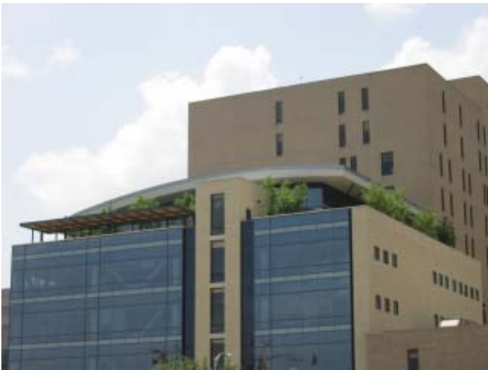
The South Texas Law School garden roof provides greenspace for employees and students as well as cooling this part of the roof structure.
