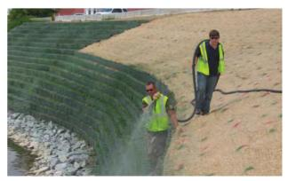
Tensar's HydraMax System can be installed three times faster than erosion control blankets with 1/3 of the man power.
